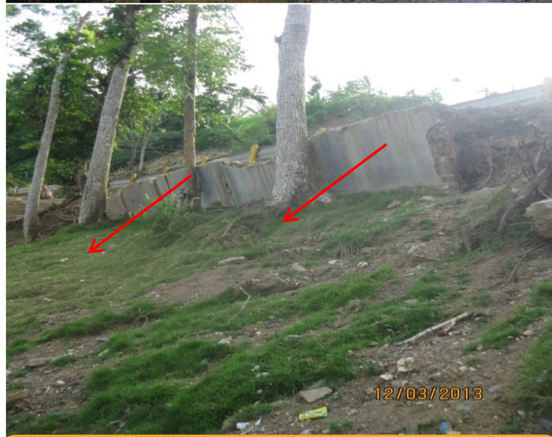
Tilting of fence/walls
