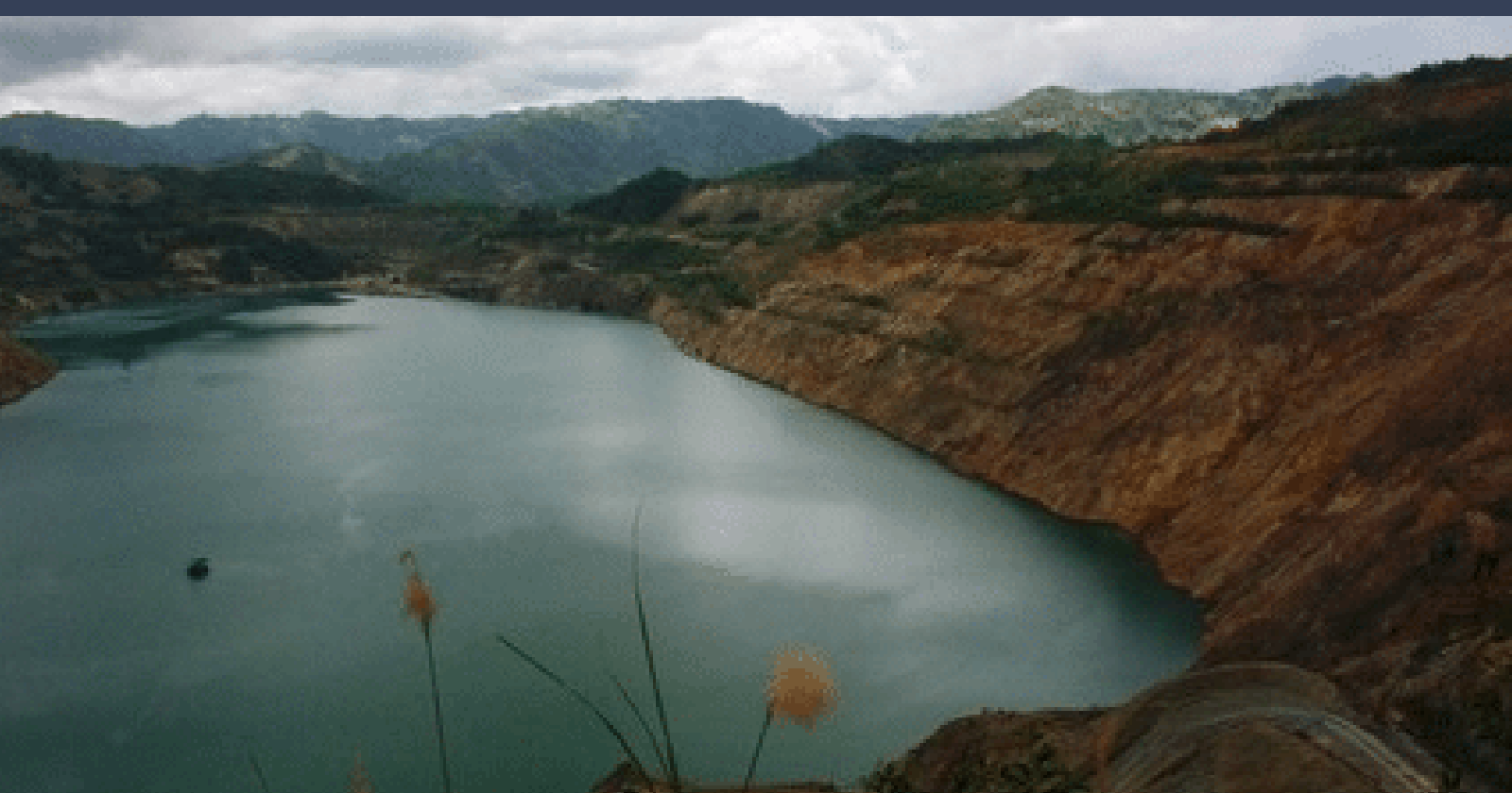
Biga Pit Tailings Storage Facility (TSF) Carmen Copper Corporation
